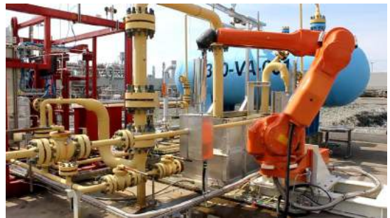
Fig. 9. The valve manipulation operation has been performed successfully tens of times on-site.
